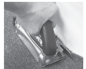
4. Using the guide bar, tuck the carpet into the gully to complete the job. The large handle will permit you to use both hands when necessary.
